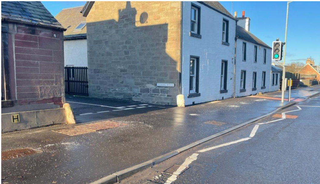
Figure 23 Continuous footway using pulled back give way markings along the School Road junction with the A94 near Burrelton Primary School © Perth & Kinross Council
